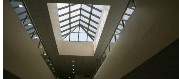
Fig. 5 On-site installation of the skylight
