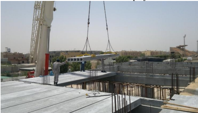
Fig. 2 Onsite installation of the HCS.
